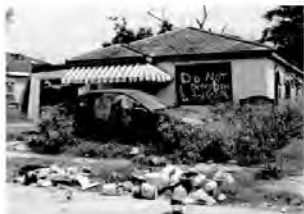
Figure 30.2 (Left) Spray-painted notice by ACORN in defence of eminent domain seizures and premature demolition by the city authorities. In June 2006 when this photo was taken, many residents had not returned because the city authorities prohibited entry to the neighbourhood until May. (Delia Wendel)
